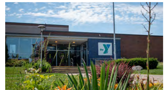
Built in 1959, the Hilltop YMCA cost $277,016 to construct ($2.7 million in 2019). Throughout the 1970s it was the weekly meeting place of the Hilltop Kiwanis before it became open to women in 1987.
