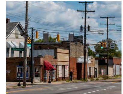
One-story commercial buildings at the intersection of Sullivant Avenue and Richardson Avenue.
