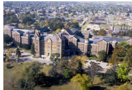
A 1989 report said lack of maintenance by the state had resulted in serious structural deterioration, with restoration costs estimated from $50-$80 million. 4
