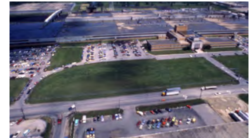
The White-Westingshouse plant employed just 300 by the 1980s, when it was sold to Big Lots liquidation stores. 4 The 175,000 sq. ft. Big Lots headquarters were located here until 2018, but the facility still serves as a distribution center today.
